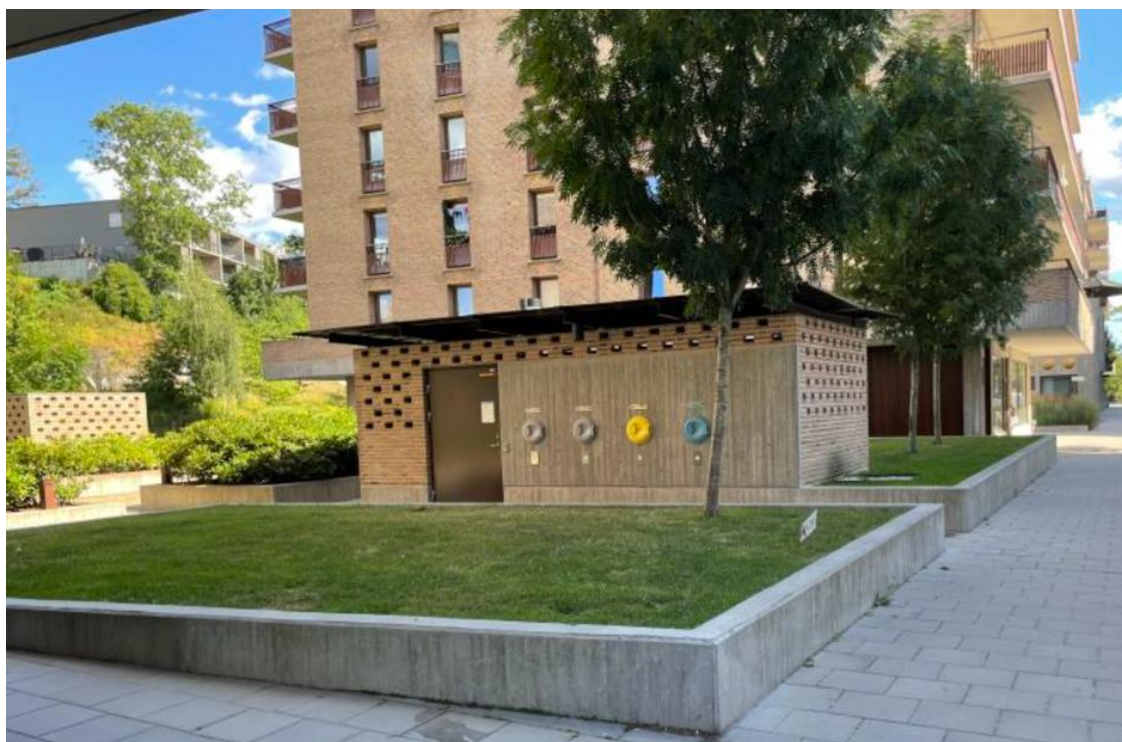
Figure 4.1 Waste house of an apartment building. Photo: OÜ Sfäär Planeeringud
